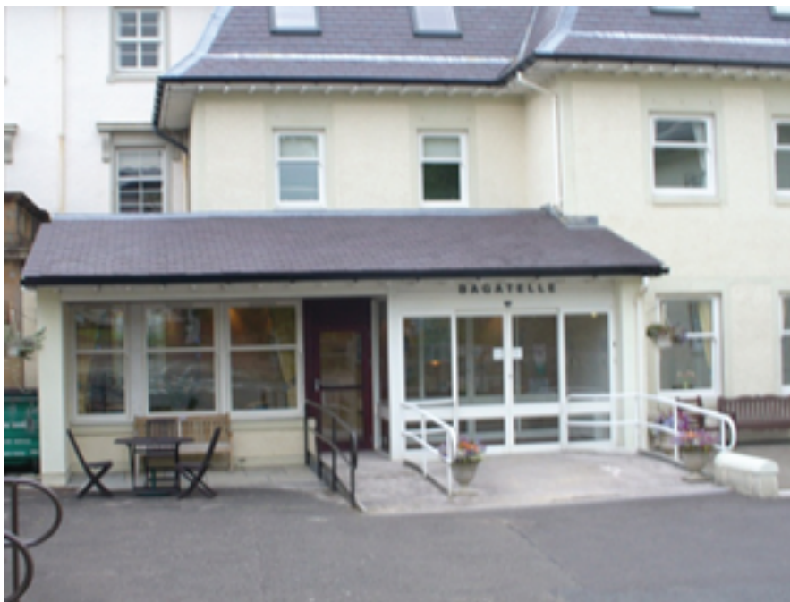
EndoTherm™ was added to the heating system at Bagatelle Care Home
